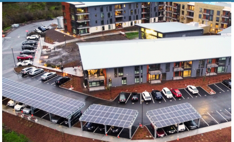
Solar panels on the resident parking area at Enso Village.
